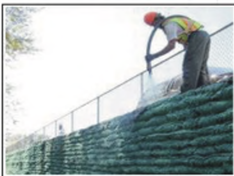
Applying Hydroseed
